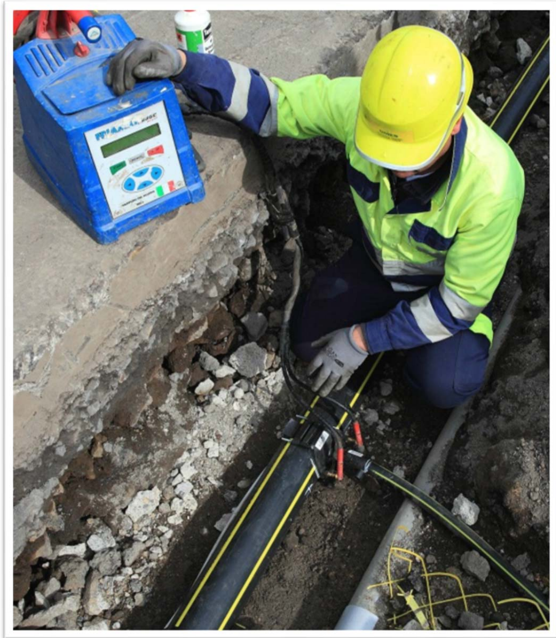
San Giovanni la Punta – Laying of the gas network
